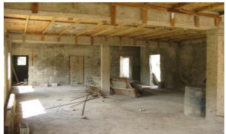
The roof/2nd floor is formed and poured.
